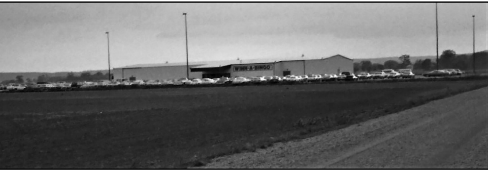
Where it all began in 1992 on April 30 th . The facility was originally a bingo parlor called Winn-A-Bingo! With gaming opportunities greatly increasing over the years, WinnaVegas Casino Resort is one of the few places in Siouxland offering bingo.
