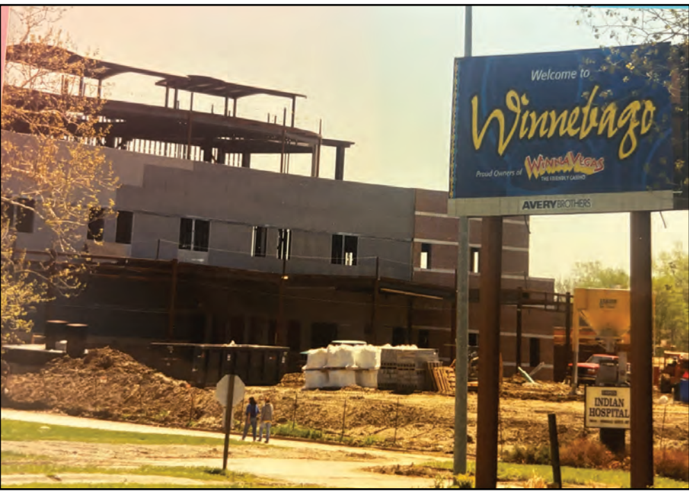
IHS Twelve Clans being constructed
