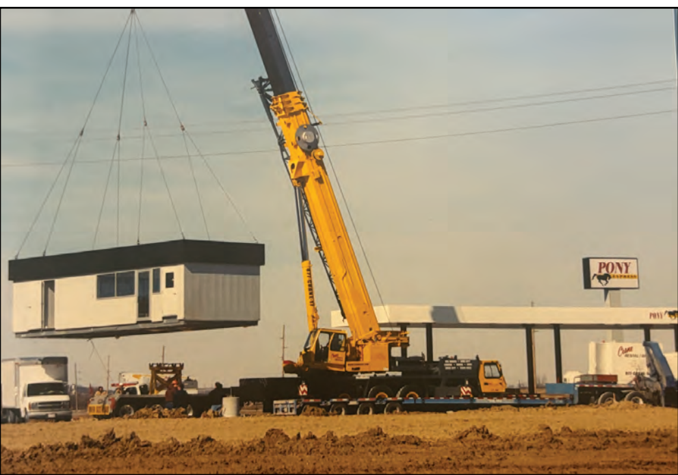
Pony Gas building being placed
