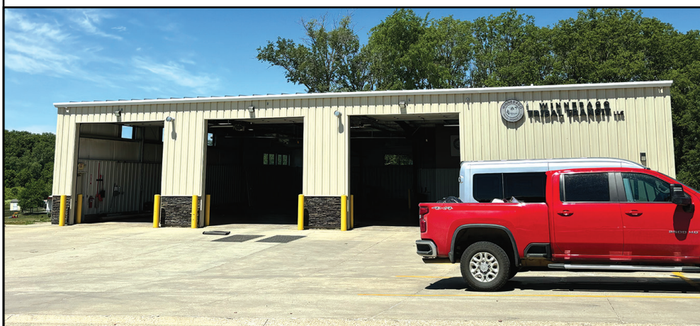
The Tribal Transit garage recently received some updates.
