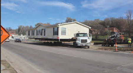
Traffic in Winnebago was almost madness last week, from the construction work along Bluff street to the transport of this house through that same construction zone. Thanks to local law enforcement officers for stepping in and directing traffic!
