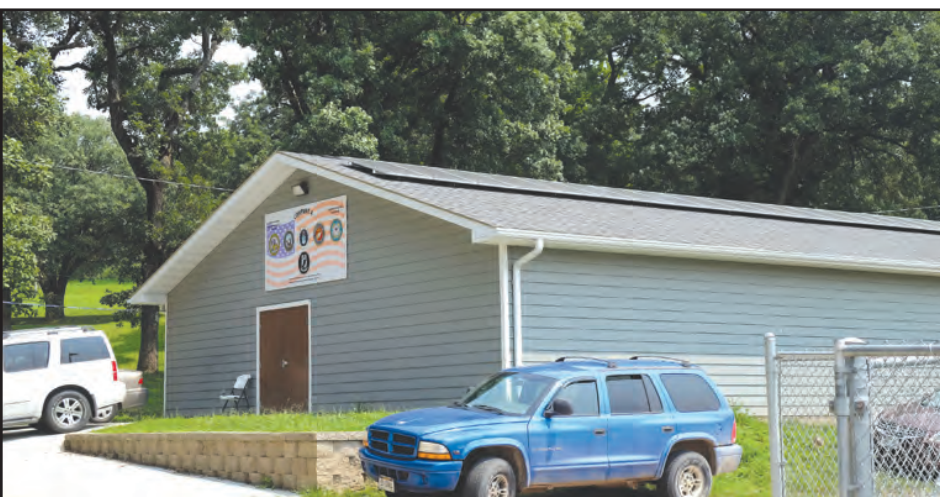
American Legion Post 363 is one of more than a dozen sites in Winnebago affixed with solar panels, which have generated significant financial savings for the community while also reducing CO2.
