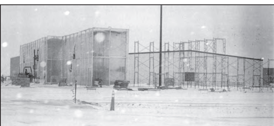
The first building for WinnaVegas while under construction.
