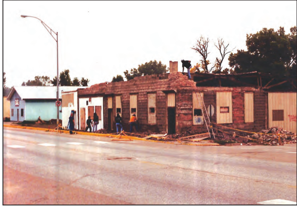
Early 90's view of the old iconic Merry Mart getting demolished
