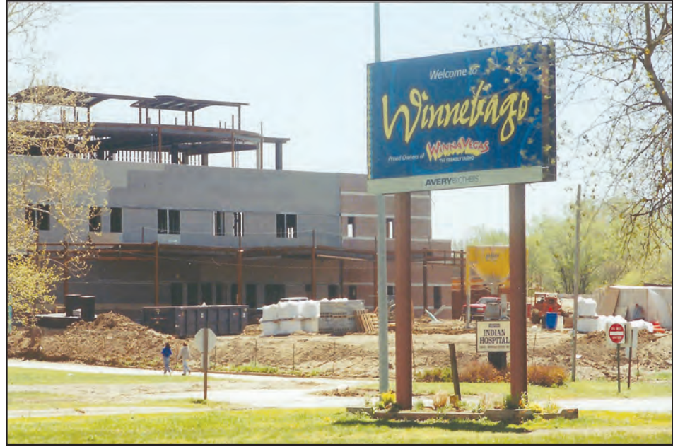
Construction of the new treaty hospital, back in 2002
