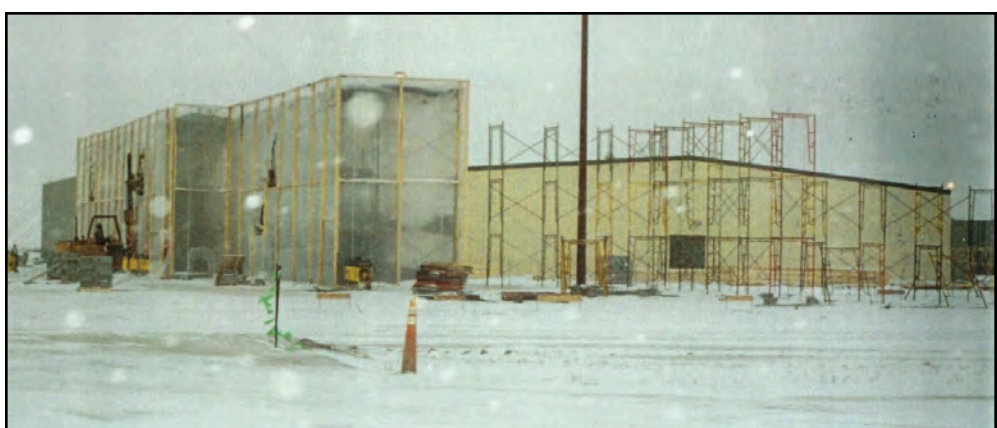
WinnaVegas Casino under construction 1993
