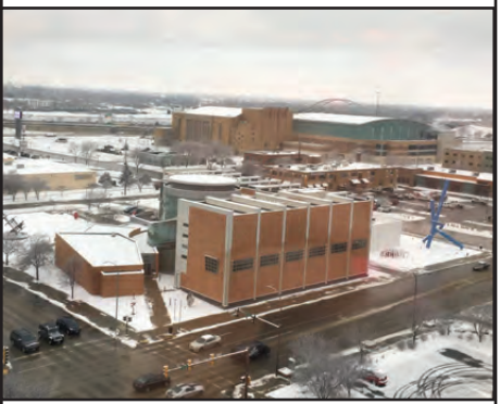
The cold weather continues... a view from the 8th floor at the HoChunk building in Sioux City, IA.
