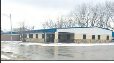
The work on the Neola Walker building is almost complete.
