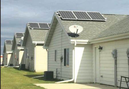
HCI has been installing Solar Panels on a number of local organizations and here on Elders Homes in the HoChunk Village.
